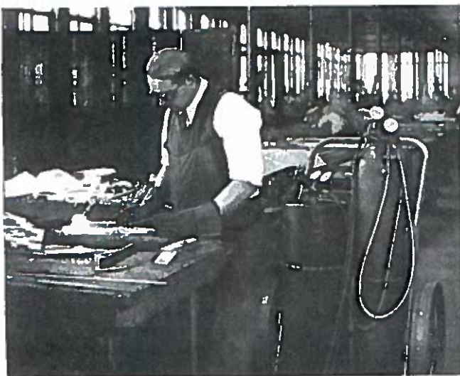
WELDING MONEL METAL WITH ACETYLENE TORCH
