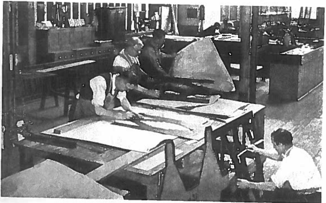
SHOP WORK ON MONEL METAL SCREEN FOR BANKING OFFICES
