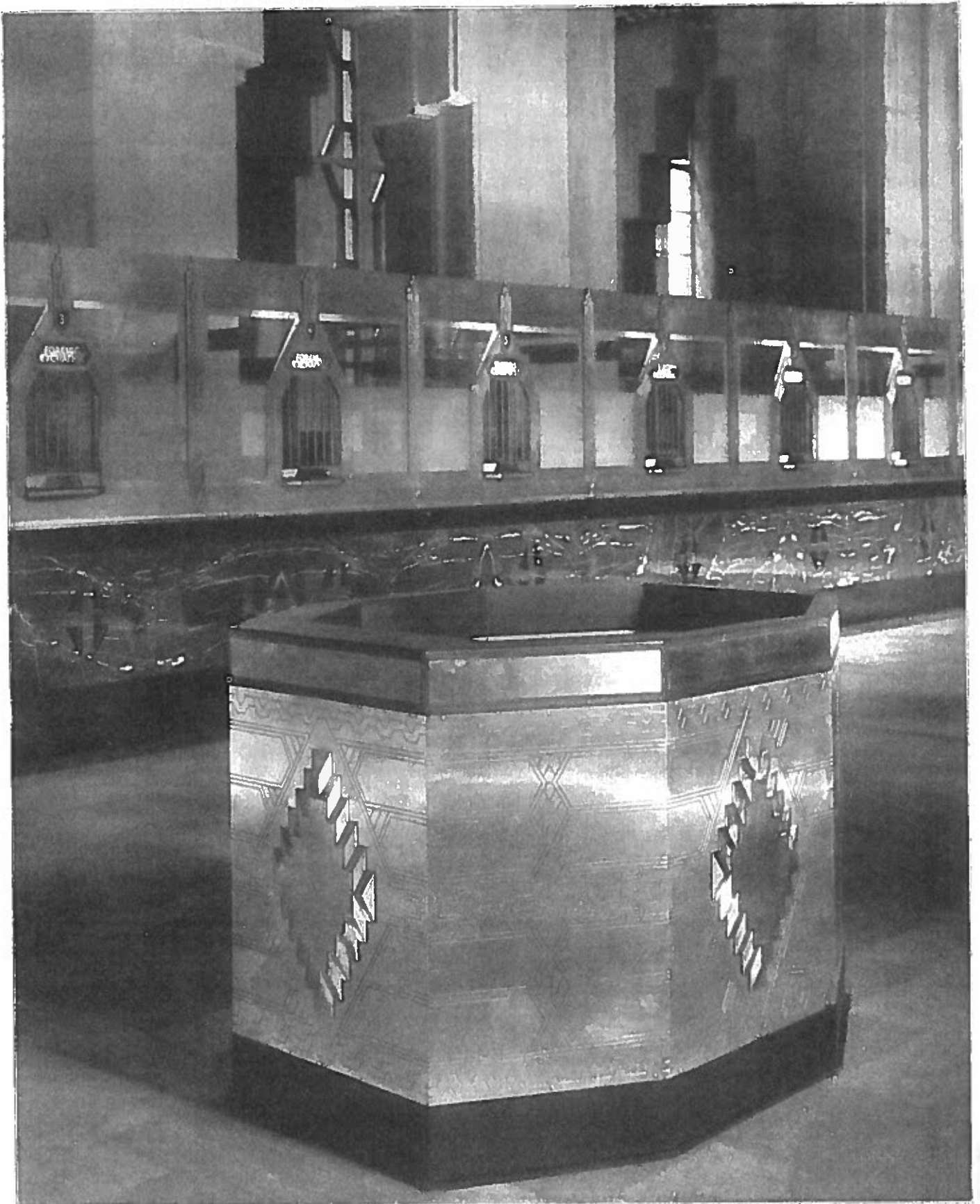
THE ESSENTIAL MODERN DESIGN IS EMPHASIZED IN THE GUARD'S STAND EXECUTED IN MONEL METAL
