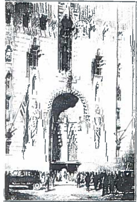
GREAT PORTAL ON GRISWOLD STREET
